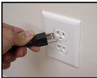
Plug the HairVac into a grounded wall electrical receptacle. Never remove the third, round ground prong. Doing so can cause a risk of electric shock.
