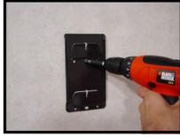
Secure wall bracket with 2 screws through the center holes on the bracket. Depending on wall type, other appropriate anchors (not provided), suitable for your particular wall type must be used.
