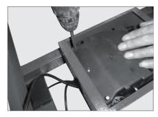
**2.** Remove the screws holding the old Control Box in place.
