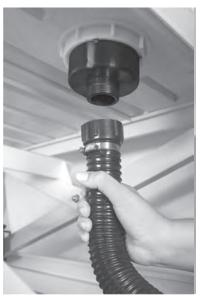
7). Attach the Hose (E) to the bottom of the Drain (F) (underneath the tub base) and screw it to secure.
