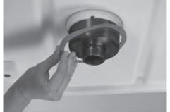
3). Underneath the base of the tub, place the Washer (I) over the bottom of the Drain (F).
